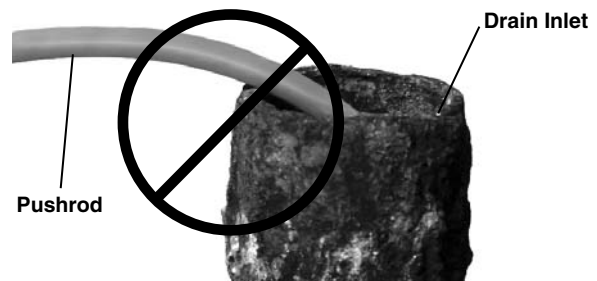
Figure 19 – Avoid Pulling At Sharp Angles
